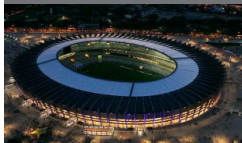
MARTIFER SOLAR Belo Horizonte / MG
