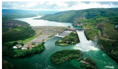
CEMIG Belo Horizonte / MG
